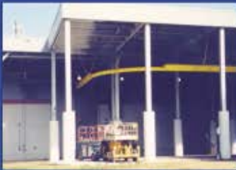
Underside of American Airlines portico protected with RC 2000.
