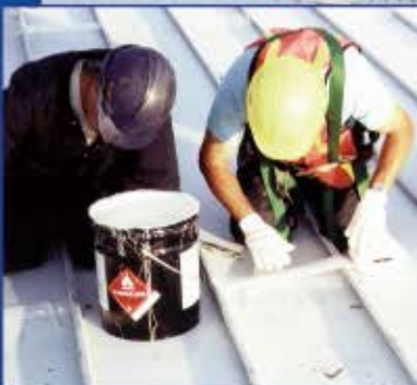
Metal roof of NATO base facility protected with Inland RC 2200 Seam Compound and RC 2000 Rubber Coating.
