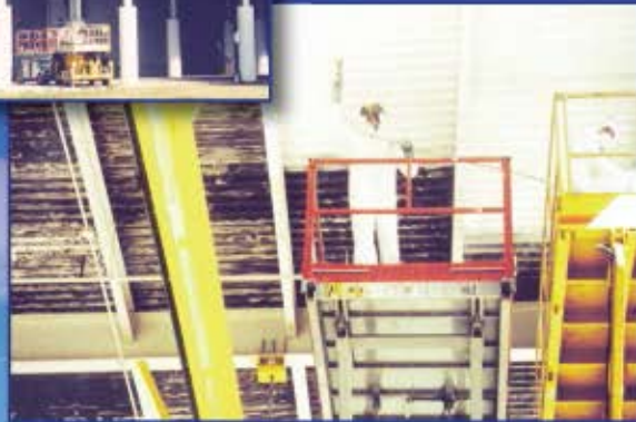
Underside of American Airlines portico protected with RC 2000.
