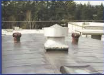
Modified bitumen roof coated with RS 2030 Sealer and RC 2000.
