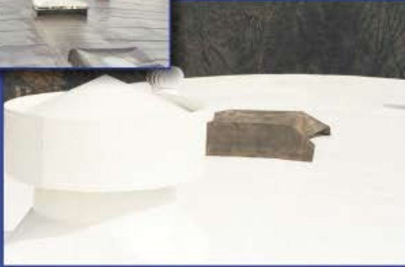
Modified bitumen roof coated with RS 2030 Sealer and RC 2000.
