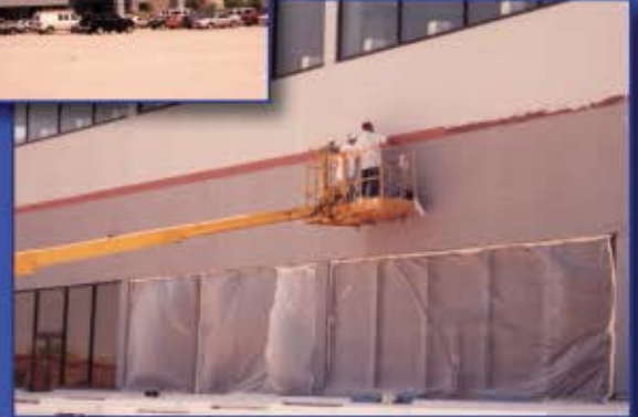
Exterior stucco surfaces of Wichita Greyhound Park coated with RC 2000.
