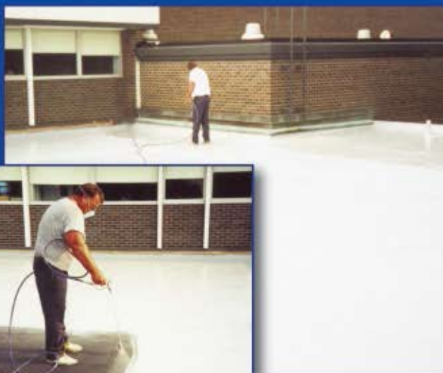
EPDM school roof coated with RC 2000 Rubber Roof Coating.
